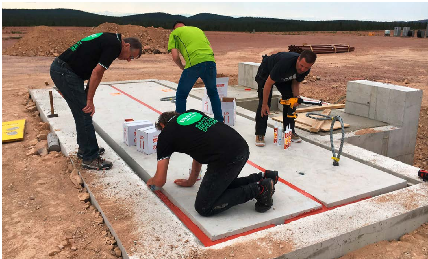
Figure 2: Installation of the joint seals.
